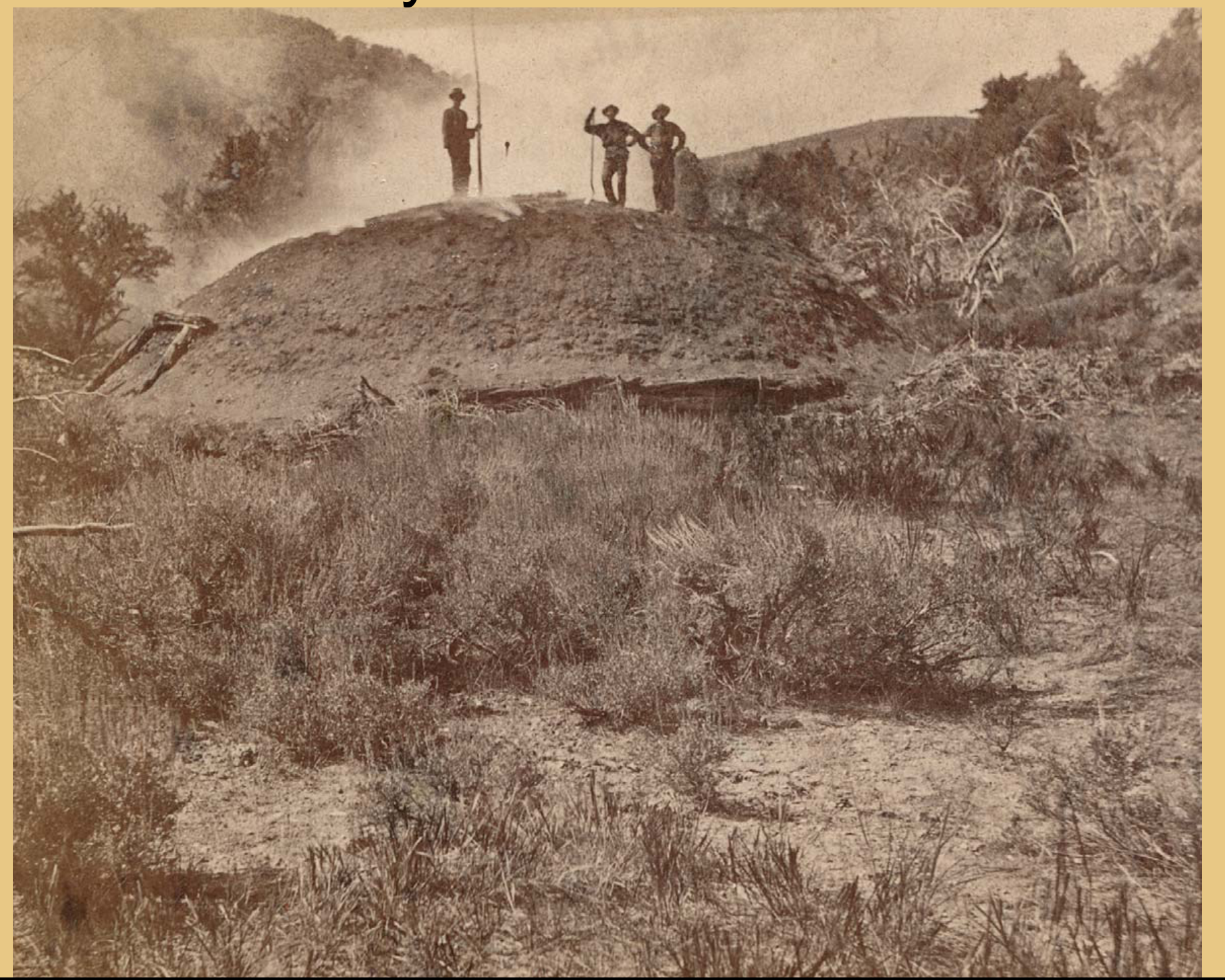
A charcoal pit in the process of burning with charcoal burners atop. (J. B. Monaco Collection [SFP 48], San Francisco History Center, San Francisco Public Library.)
